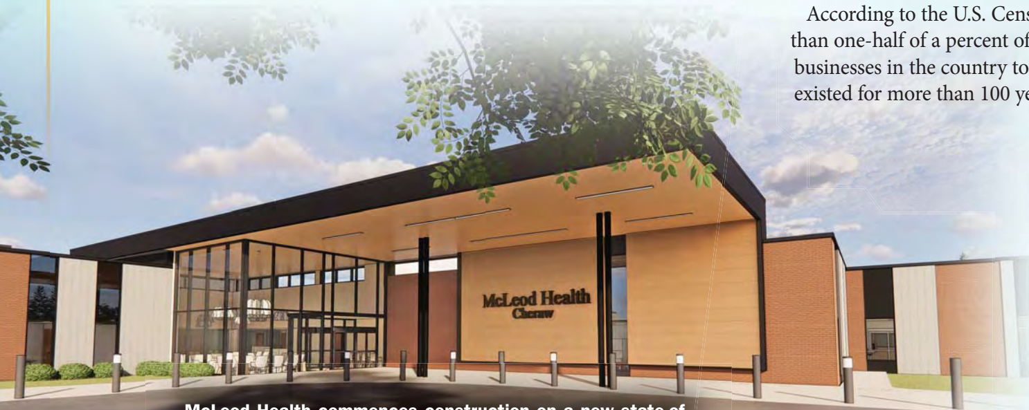
McLeod Health commences construction on a new state-of-the-art expansion of McLeod Health Cheraw in 2026.
